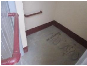
Handrails placed inside the door and on the wall
