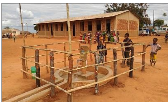
Borehole with hand pump constructed in the Project
