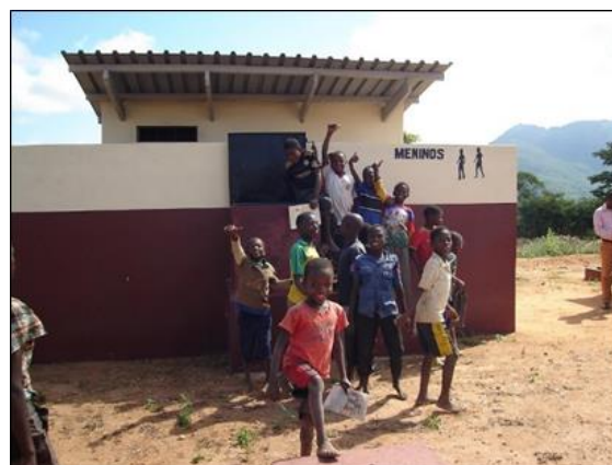
School latrine (for boys)
