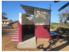
Slope at the entrance
